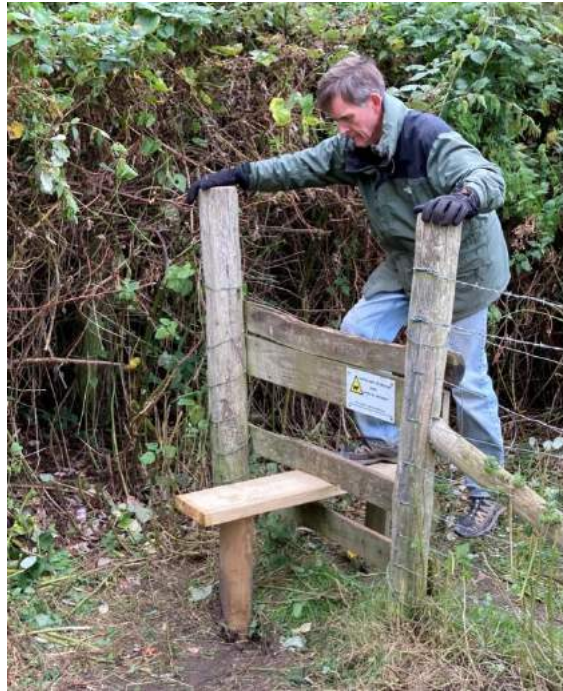
Vegetation cut back and stile renewed
