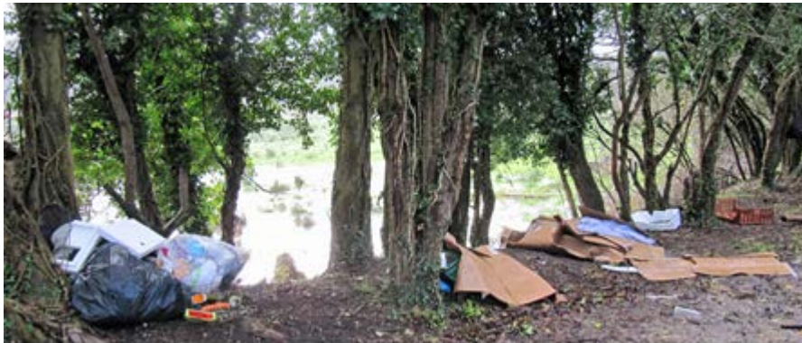
litter left by campers on the embankment
