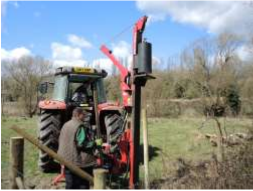
posts for fencing
