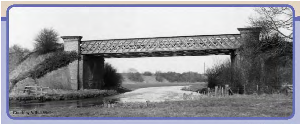
original Elham Valley line bridge
