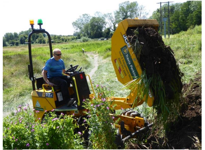
Dumping the spoil by the railway fence
