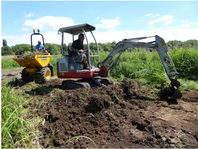
Starting to dig out the pond
