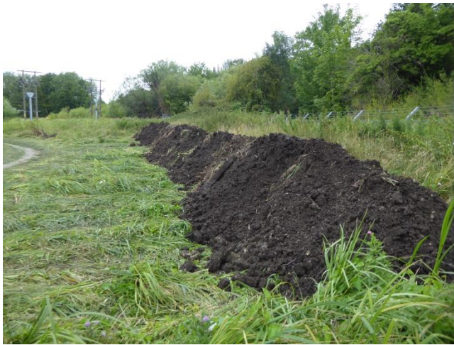
Spoil heap before grading and flattening
